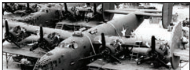
During WWII, Rohr designed and produced over 35,000 engine installation packages, consisting of mounts, cowlings and accessories for the Navy PB2Y Coronado and Air Force.
