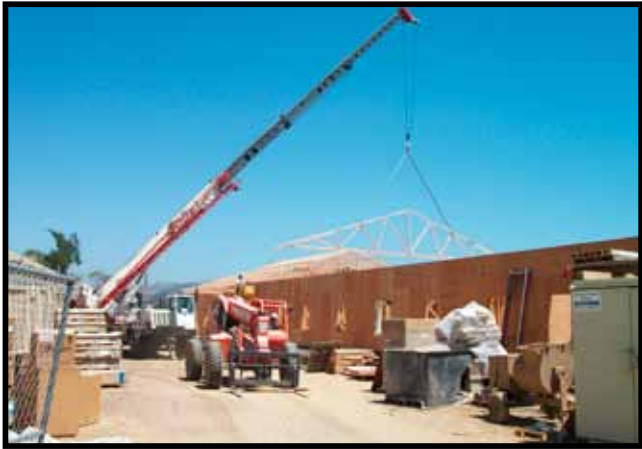
Bob Turner's Crane Service (Lakeside Contractor) lifting a joist for the second level of the new fire station.. Photo credit: Patt Bixby
